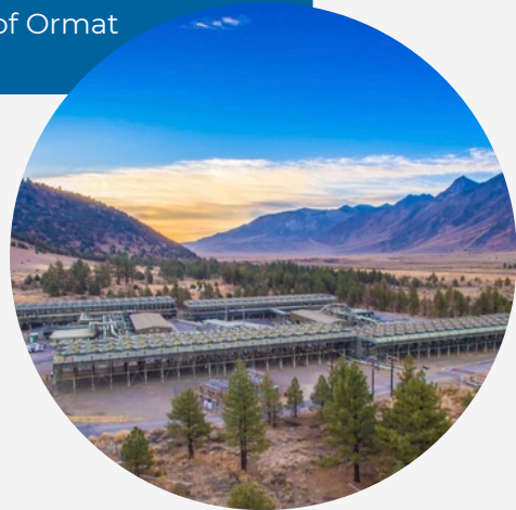
Ormat Mammoth 2 Geothermal Facility
